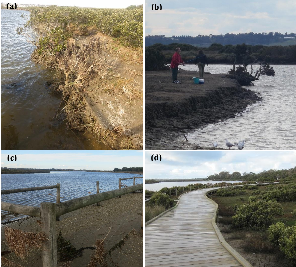
Figure 7. a) Eroding banks are present along much of the inner section of the Barwon River estuary with b) fisher-people commonly observed walking along banks and likely contributing to the problem. It appears as though a number of different methods of protection have been trialled, including c) fencing off particular sections of mangroves (which in this case are no longer present), or d) creating boardwalks
